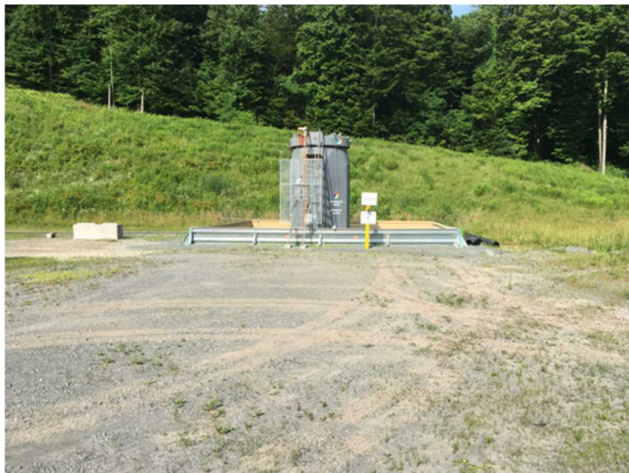
Photo #2. Truck tire tracks indicating Vac Trucks common route to back into remove produced water and rain water from secondary containment.
